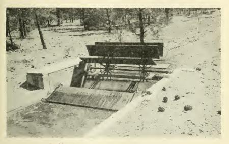
Looking downstream on a parallel bar fish screen Cleaning bar on screen just above water
